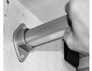
9. Partially fasten second flange to wall using **ONE** screw. Carefully position wires into one of the grooves located on back of flange. Secure flange to wall with remaining screw, making sure wire is in flange groove. (If wires come through drywall and into the fixture, this step is not needed.)
