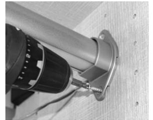
10. Push rod against the wall in "non-wired" flange and tighten the set screw.
